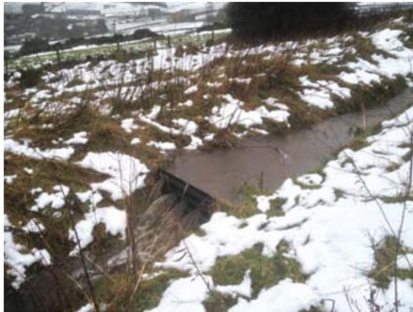
Experimental plate weirs used for water storage and slowing the flow.
